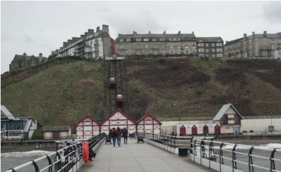
Saltburn-by-the-Sea cliff lift, 22/2/2024
