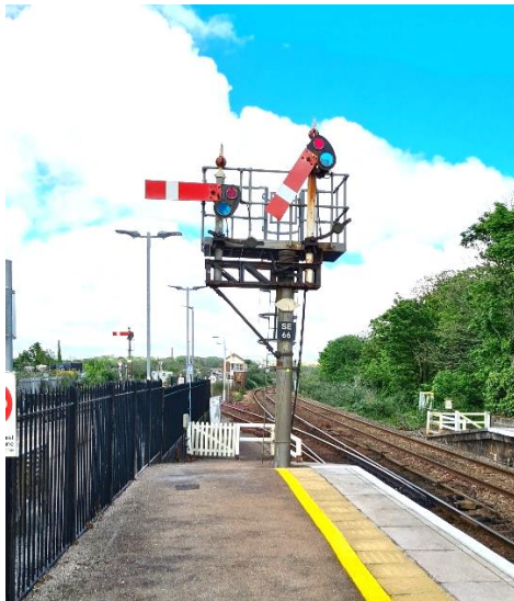
Lower-quadrant signals still in use at St Erth, Cornwall, photographed on 15/5/2024.
